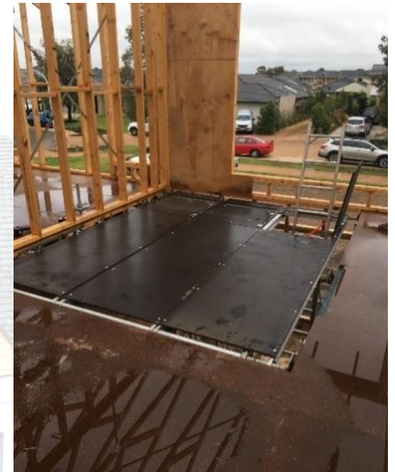
Void Protection and Access
